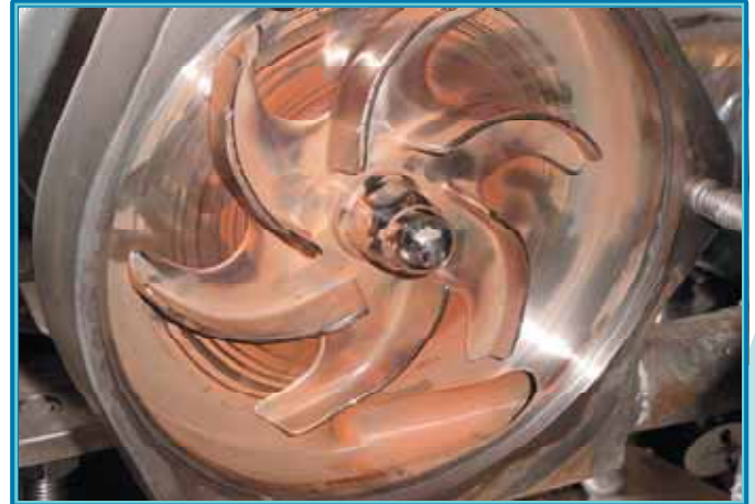
Rouging Identified During a Honeyman Site Survey
